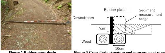
Figure 2 Rubber cross drain
