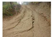
Figure 1. Operation road where the surface was eroded
